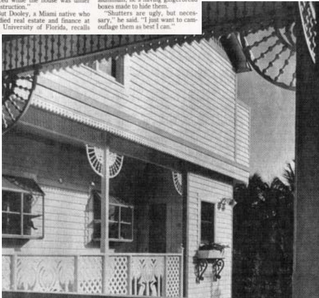
GOOD OLD DAYS: The home's gingerbread scrolls used in doorways and on porches were bought from Cumberland Wood Craft Co. in Durango, Colo. A tin roof, shingled exterior trim and beveled, etched windows add to the look. The home's hurricane shutters will have gingerbread boxes to camouflage them.
